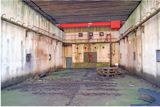
Internal view of K2. Note the high-speed camera positions in the side walls and the three elevated camera positions at the rear
